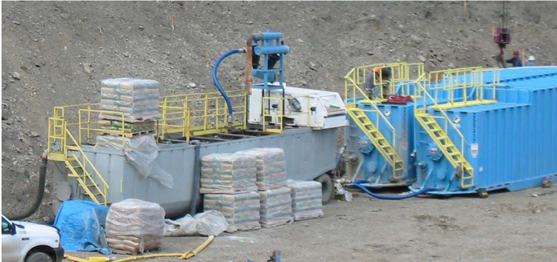
Figure 5-28 Mixing plant and holding tanks for bentonite slurry preparation
