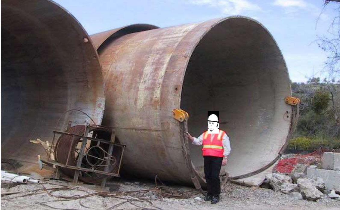
Figure 5-4 Exceptionally Large Temporary Casings
