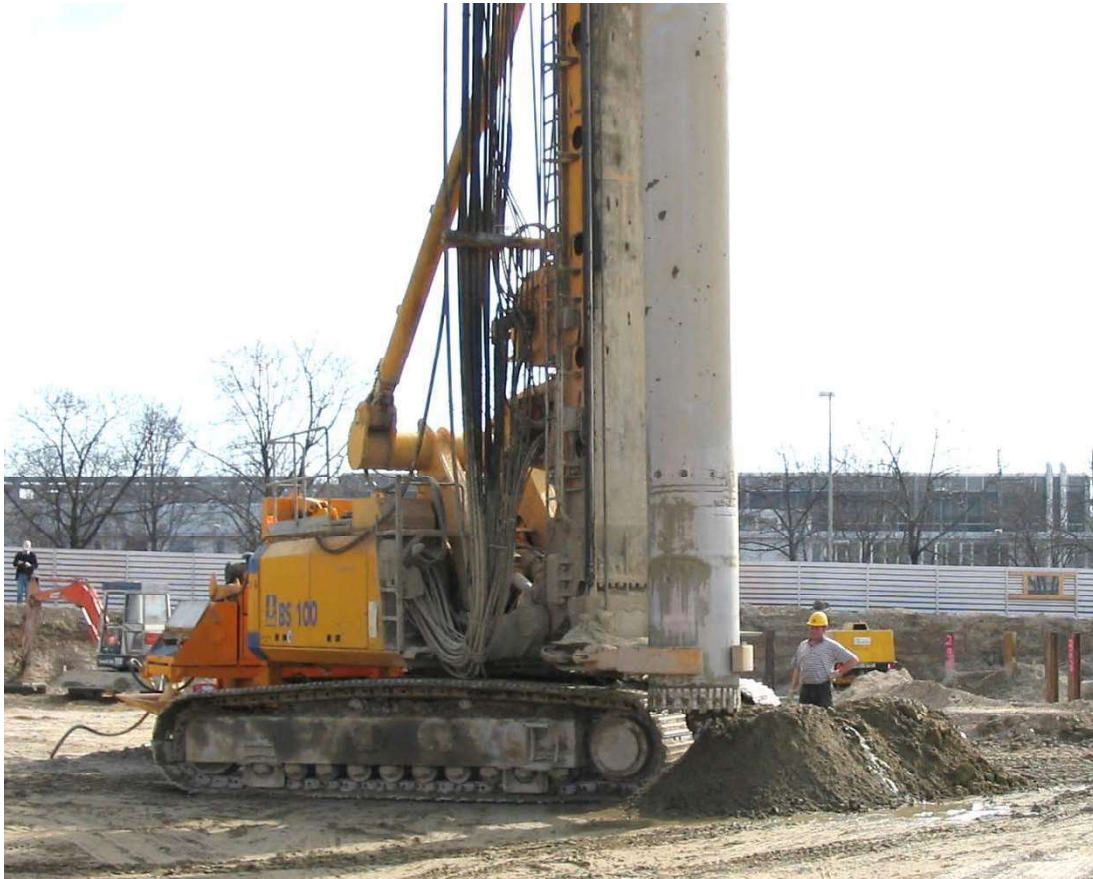
Figure 5-12 Segmental Casing Installed with a Hydraulic Drill Rig
