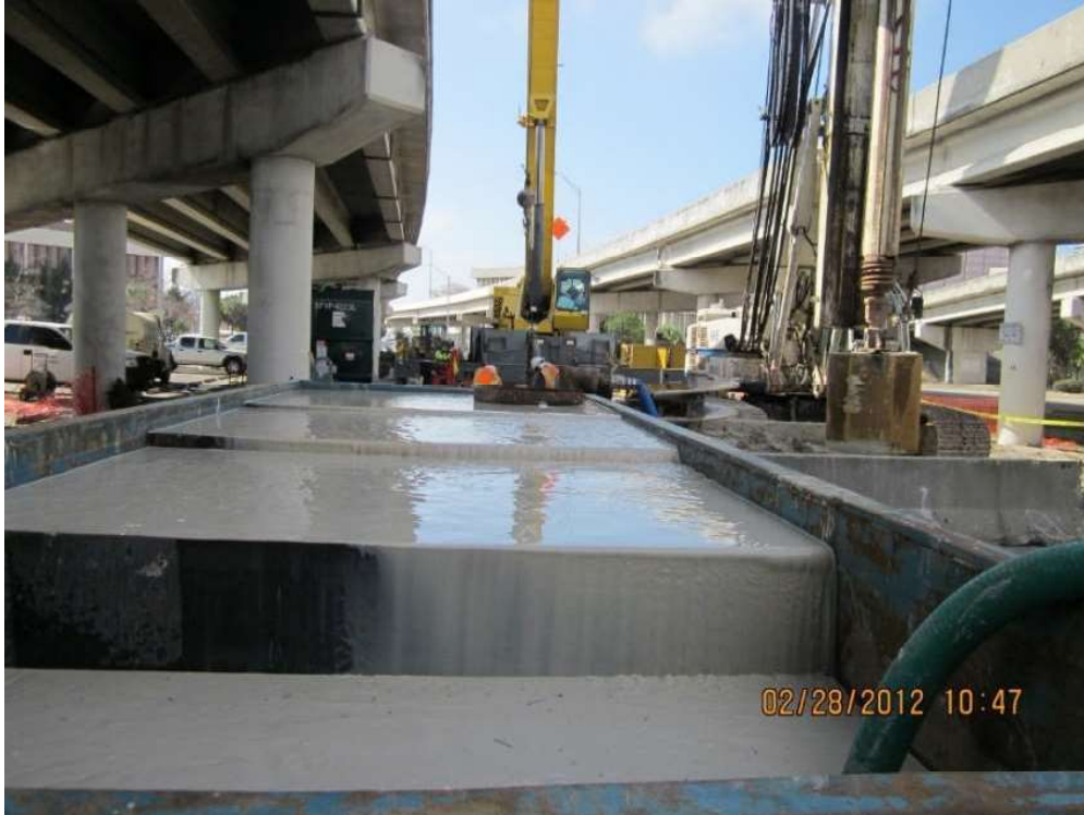
Figure 5-33 Sedimentation Tanks for Polymer Drilling Fluid
