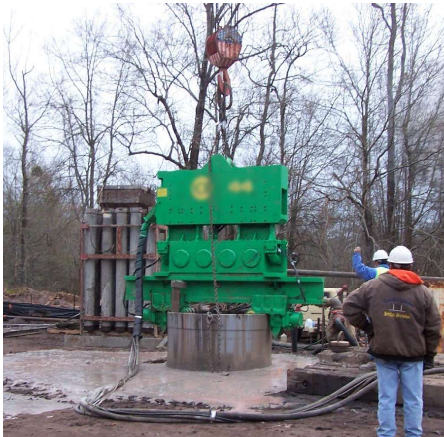
Figure 5-11 Extraction of Temporary Casing Using a Vibratory Hammer
