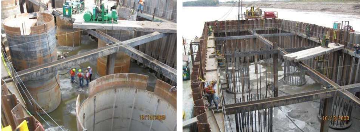
Figure 5-19 Permanent Casing Used for a Shaft Group Foundation in a River
