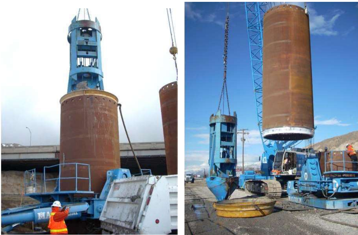
Figure 5-5 Segmental Casing Installation with Oscillator System
