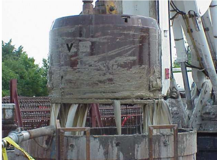
Figure 5-25 Mineral Based Drilling Fluid (Bentonite Slurry)
