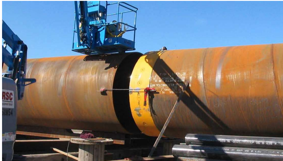
Figure 5-6 Installation of Casing Joint on Standard Pipe
