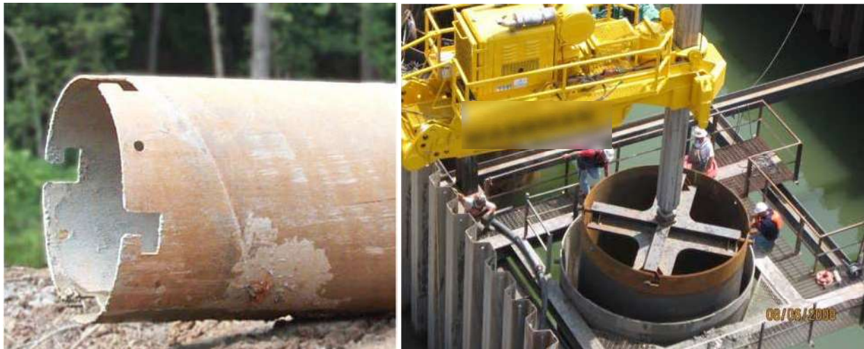
Figure 5-7 J Slots in Top of Casing for Use with Casing Twister
