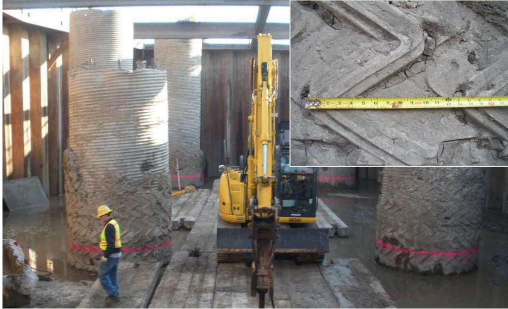
Figure 5-16 Exposed Surface of Drilled Shafts Constructed Using Oscillated and Rotated Casing
