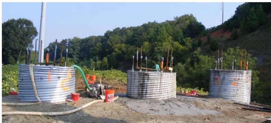
Figure 5-20 Corrugated Metal Pipe (CMP) Used as Permanent Liner
