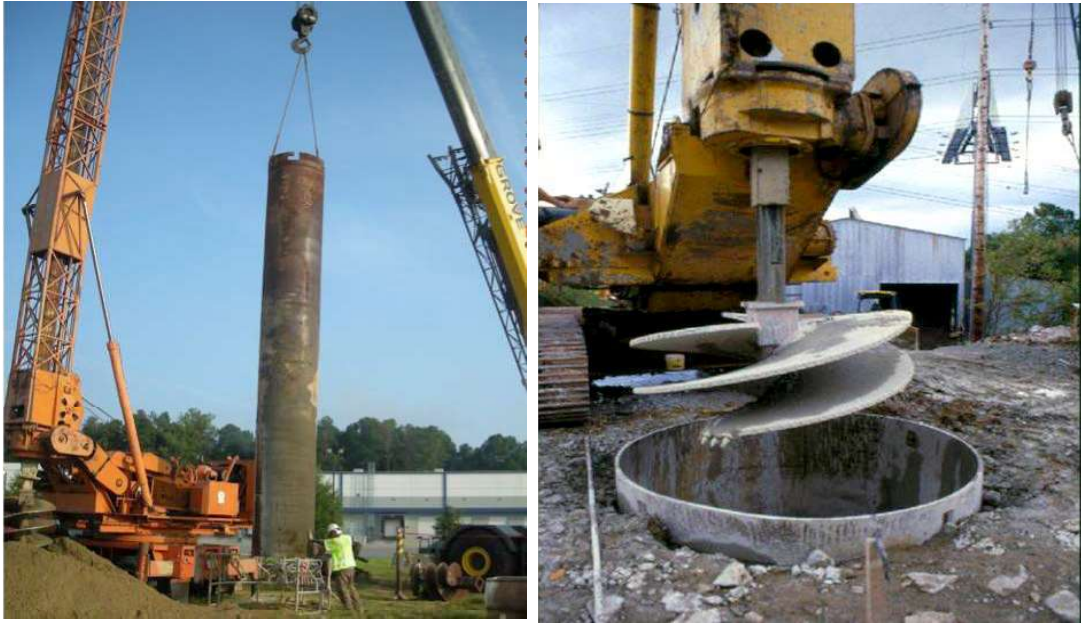
Figure 3-6 Drilling into Rock through a Cased Hole
