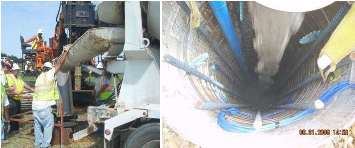
Figure 3-4 Free-fall Concrete Placement in a Dry Hole
