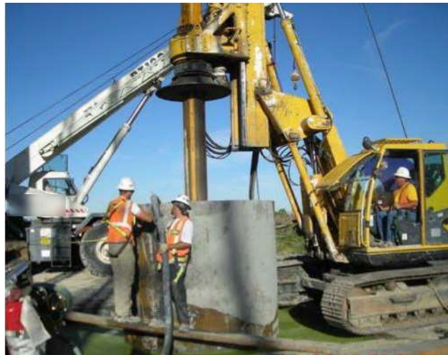
Figure 3-12 Elevated Surface Casing to Provide Fluid Head Above Artesian Groundwater
