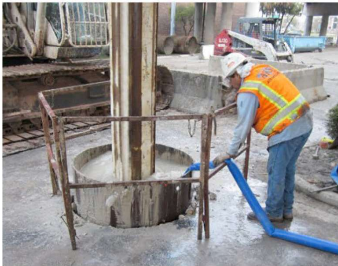
Figure 3-10 Maintaining Positive Fluid Head Pressure in the Drilled Shaft Excavation
