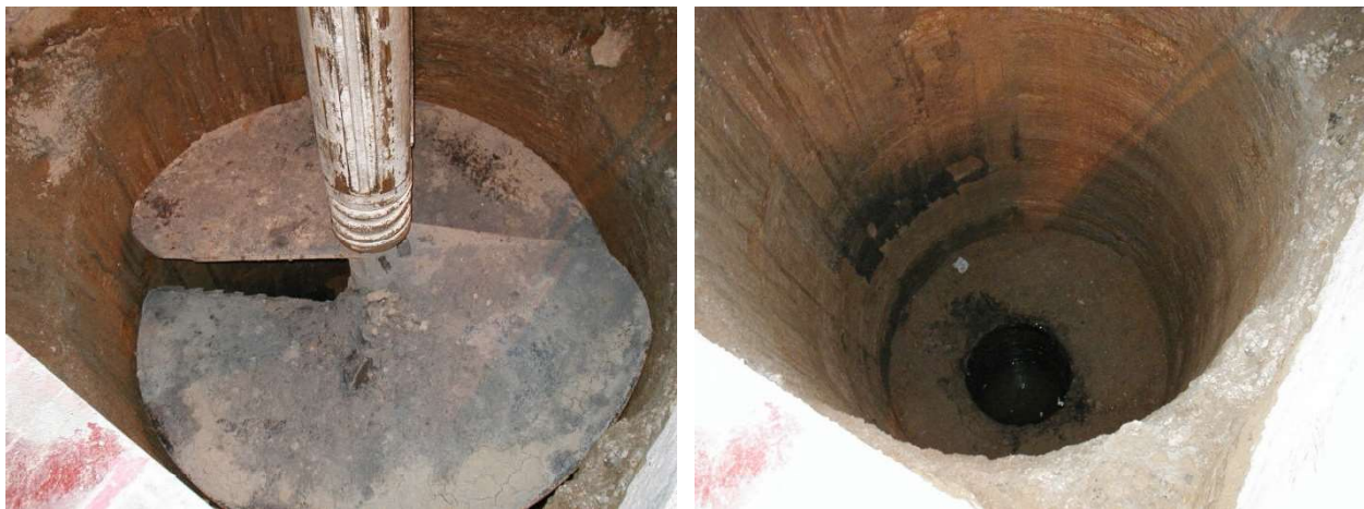
Figure 3-1 Excavation of a Drilled Shaft in Naturally Stable Soils
