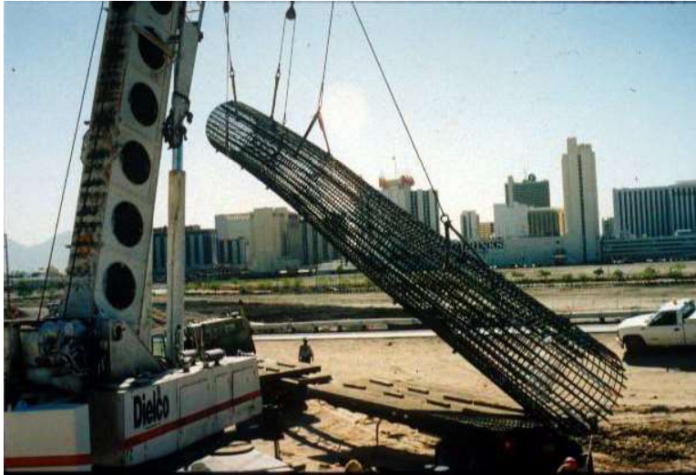
Figure 3-3 Lifting and Placing the Reinforcement
