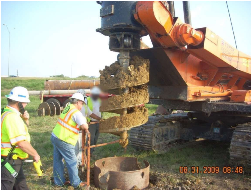
Figure 3-2 Visual Inspection of Excavated Materials for Construction Records
